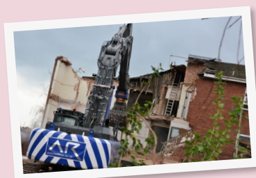
Right: Demolition of the former Woodside home is almost complete...
